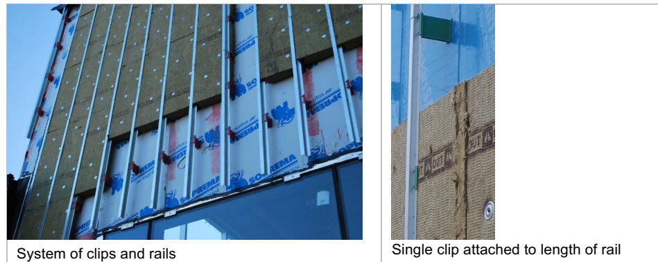
Figure 2. Visual representation of Cascadia Clip® fiberglass thermal spacer support system
